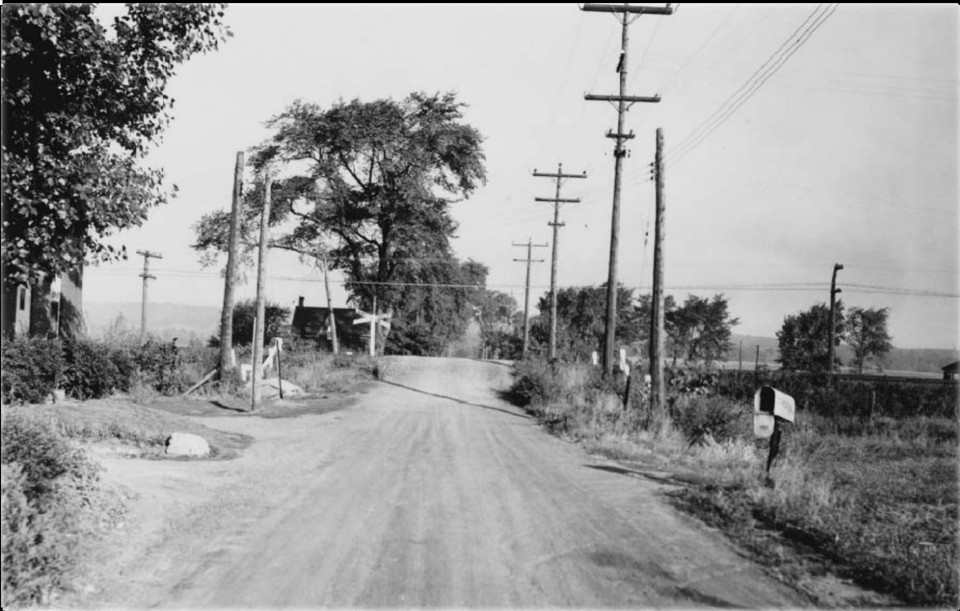
King Road North at CNR tracks
